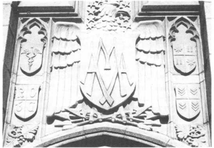
The AMA Shield above the gymnasium entrance
